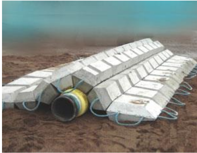
Figure 2.6: Concrete mattress of the type to be used for pipeline protection
